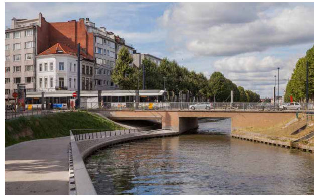
Figure 3. Underpass Rozemarijn bridge ©City of Ghent
